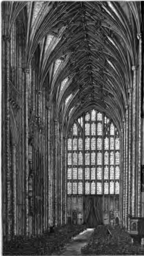
Winchester Cathedral—Nave, looking west.
